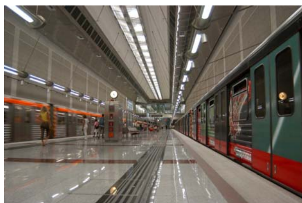
Fig. 2 Athens Metro station "Aghios Dimitrios"
