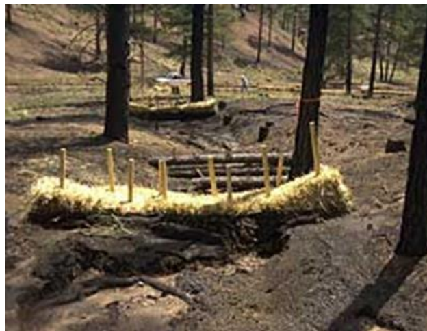
Fig 6 - Channel treatment with logs and straw bales barrier.
