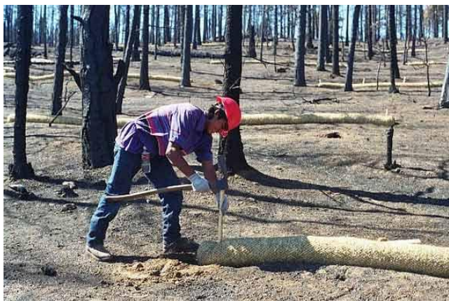
Fig 5 - Contouring made with straw wattles. Source: Forest Service, USDA
