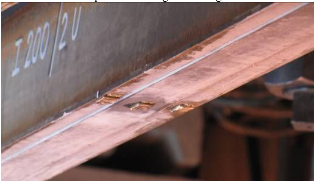
Fig. 6 strain gauges on bottom flange of steel beam and on CFRP
