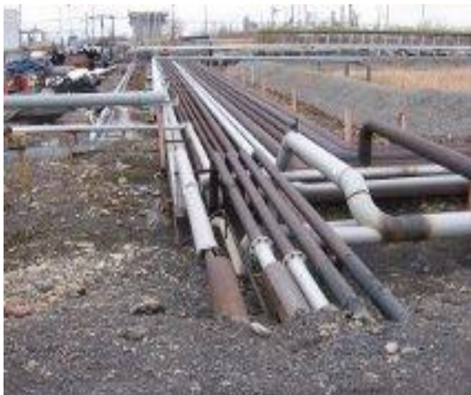
Fig. 4: One research site: some prefabricated pipes after their installation
